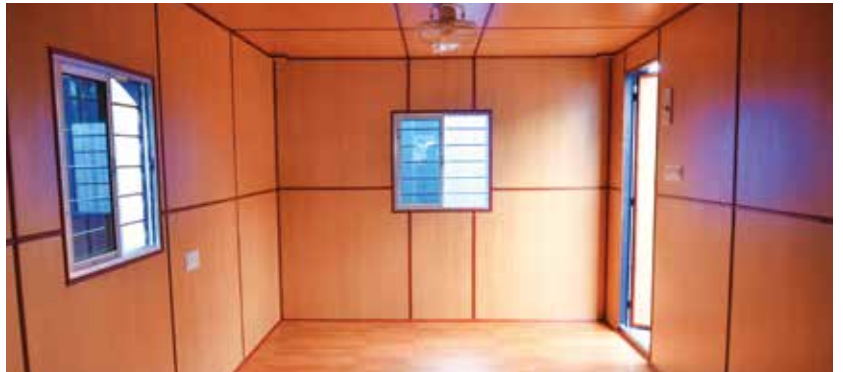
General site office
